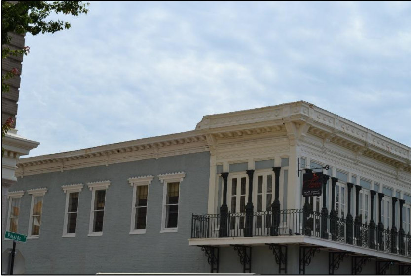
The Classical Revival details on this building are concentrated on its primary, Palafox-facing elevation. The simpler sash windows and lintel ornamentation are located on a secondary elevation, which faces Romana Street.
