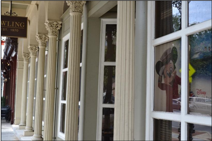
Classical, cast-iron columns in the Palafox Historic Business District.
