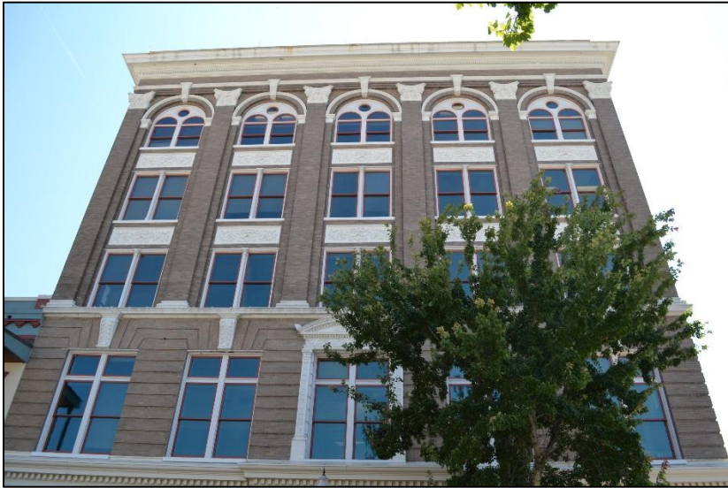
The Thiesen Building on Palafox Street is an excellent example of Renaissance Revival Architecture. Note the Classical elements, such as the column capitals and pedimented window (bottom center); the cornice detail with modillions and frieze bands add heavy, horizontal divisions to each floor.
